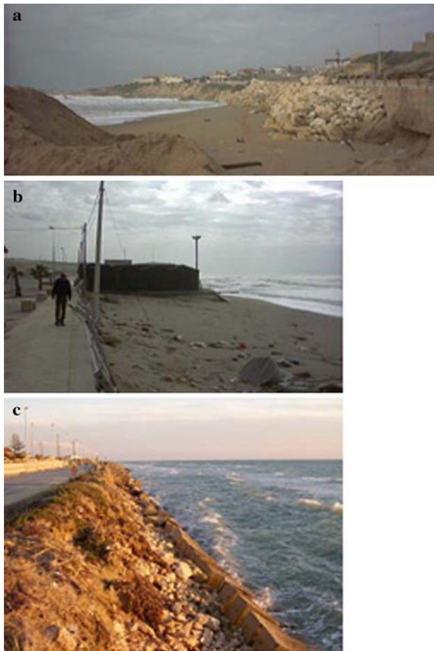
**Fig. 7** Erosive processes southward of Scoglitti breakwaters, undermining the littoral road (a), where a rip-rap revetment was created to stop cliff retreat, and a bar constructed on the dry beach (b). Concrete blocks implemented at Santa Maria del Focallo to protect the littoral road (c; photo courtesy of G. Pisana). It is possible to note wave reflection processes on the concrete blocks which produced the deepening of the nearshore zone close to the structure
