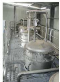
Liquid distribution system with integrated CIP cleaning nozzles.
