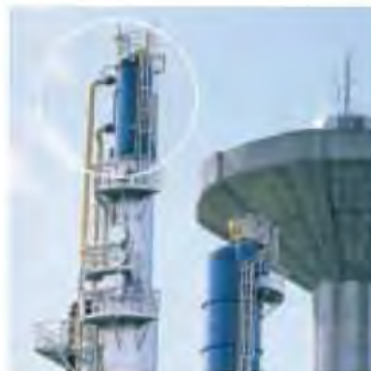
Direct mounting of a spiral condenser at a stripper tower reduces installation costs, increases product recovery and reduces pollutant escape.
